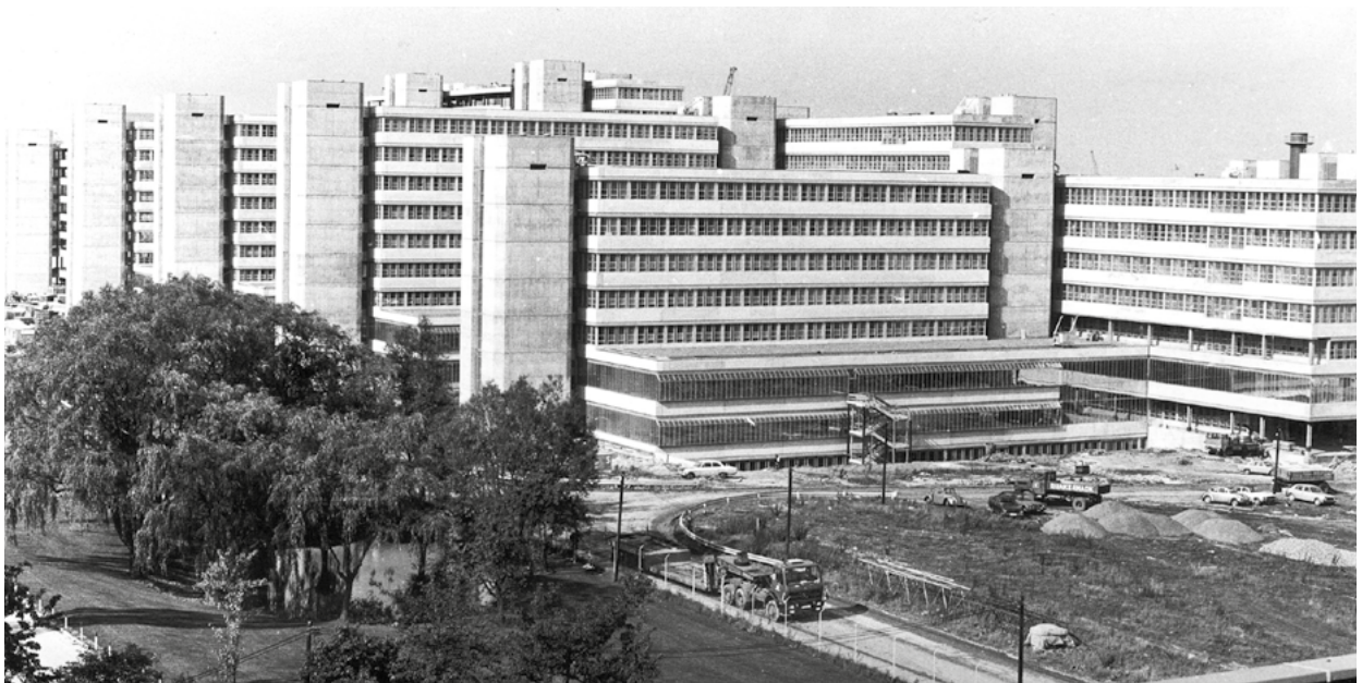
Around 1970: The Bielefeld University building.
