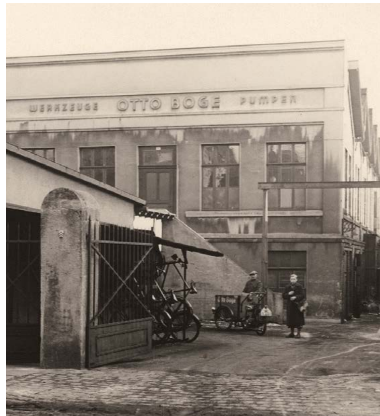
Factory building in Siechenmarschstrasse: Boge headquarters from 1921 to 1937.
