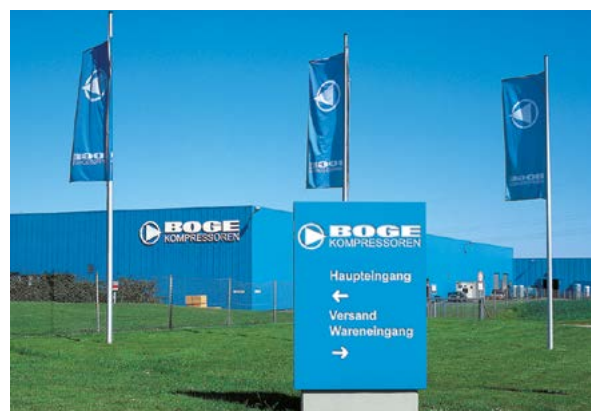
The current Boge production site in Bielefeld-Jöllenbeck.
