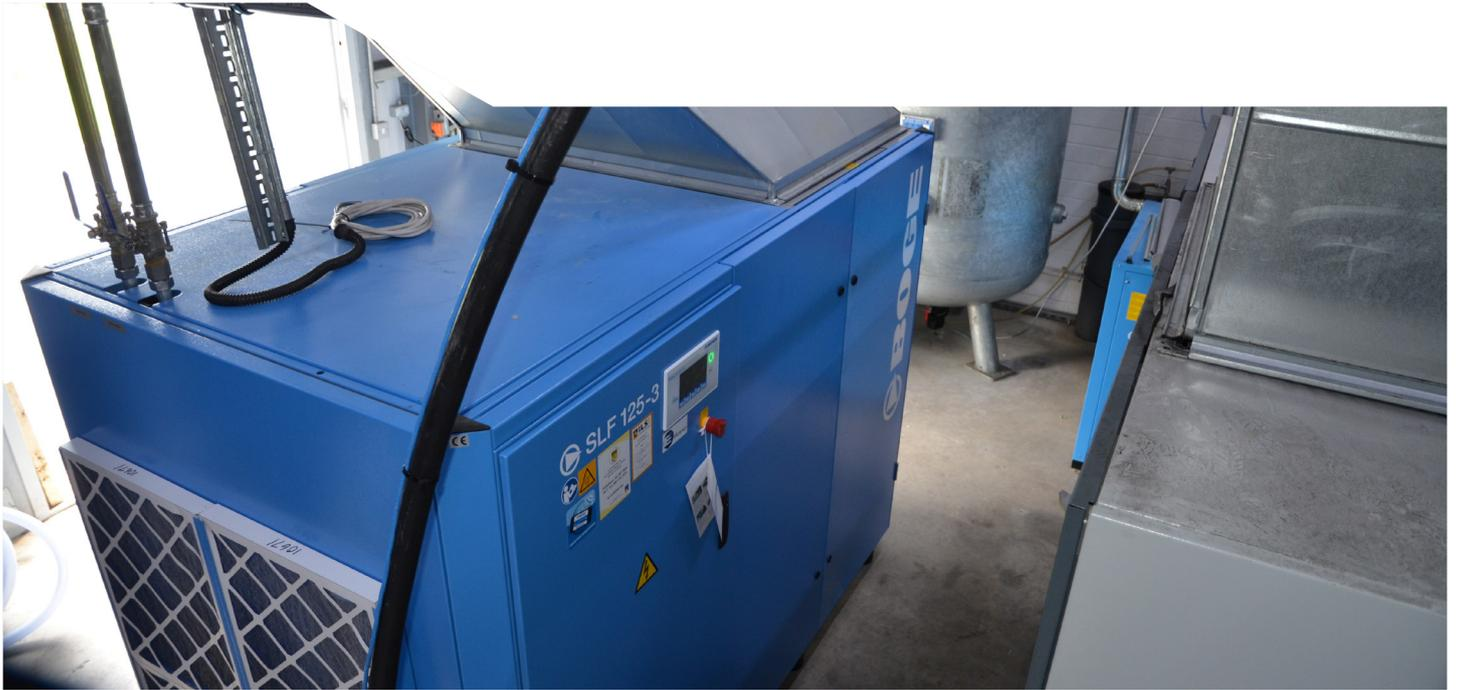
Installation took just two days and was completed during the Christmas break with no interruption to production. The old duty compressor has been retained as a standby, while the old standby will also be available for use.
