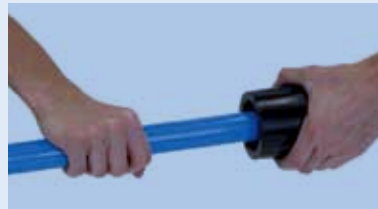
CHAMFERING Chamfer the external part of the tube in order not to damage the sealing ring.
