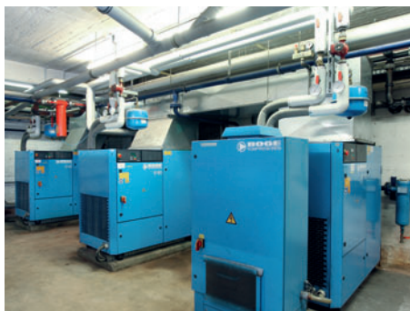
Two S 60 oil-injected screw compressors and a frequency controlled compressor from the SF 61 range provide the required compressed air.
