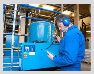
creates a tiny sound that is inaudible to the human ear – but detectable by specialist ultrasound detection equipment, which converts it into an audible signal and indicates it optically. Once leaks have been identified, a maintenance schedule must be put in place to plug them and ensure future leak detection surveys are carried out – or the benefits will only be temporary.
